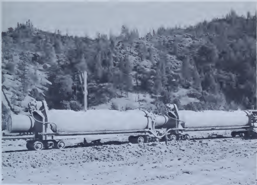
Figure 115.—Horizontal agitators used for transporting concrete for Clear Creek Tunnel, Central Valley project, California. 214-TD-4115-CV.
